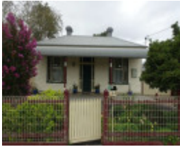
St John s Church of England Vicarage - facade
