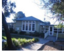
Clyde Primary School - south west view
