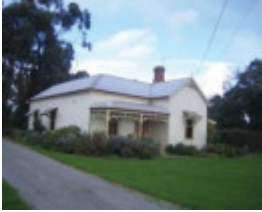
10 Ballarto Road - north east view
