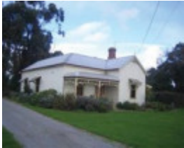
10 Ballarto Road - north east view
