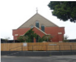
St Agatha s Catholic Church - High Street elevation facade
