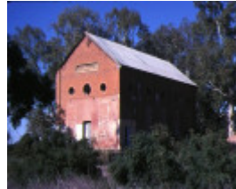
billabong pumping station nichols point irymple mildura rear view jun1982
