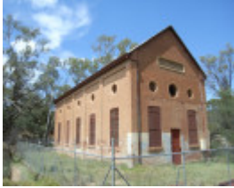
BILLABONG PUMPING STATION SOHE 2008
