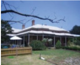
Wilandra - North East View
