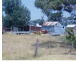
Fernlea - former dairy and machinery sheds
