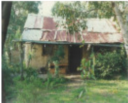
Cottage Toilet Building Henley Rd_04 - Shire of Eltham Heritage Study 1992
