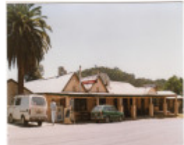
St Andrews Hotel Palm KangGround St Andrews Rd Colour 1 - Shire of Eltham Heritage Study 1992
