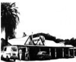
166 - St Andrews Hotel Palm KangGround St Andrews Rd 07 - Shire of Eltham Heritage Study 1992
