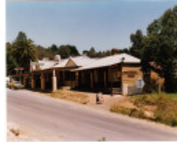
Shop Residence St Andrews Colour 3 - Shire of Eltham Heritage Study 1992
