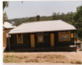
Shop Residence St Andrews Colour 2 - Shire of Eltham Heritage Study 1992
