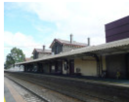
KYNETON RAILWAY STATION COMPLEX SOHE 2008
