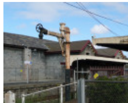
KYNETON RAILWAY STATION COMPLEX SOHE 2008
