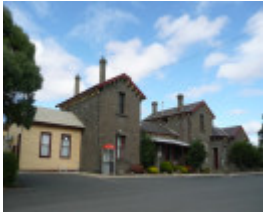
KYNETON RAILWAY STATION COMPLEX SOHE 2008
