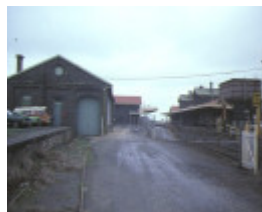
railway station goods shed & water tower station street kyneton property view sep1984
