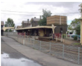
Kyneton Station North View
