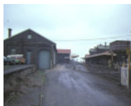
railway station goods shed & water tower station street kyneton property view sep1984
