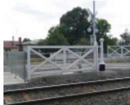
KYNETON RAILWAY STATION COMPLEX SOHE 2008
