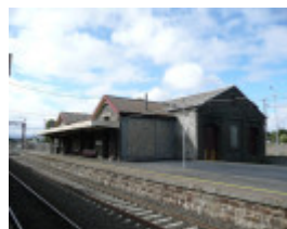
KYNETON RAILWAY STATION COMPLEX SOHE 2008
