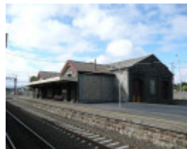
KYNETON RAILWAY STATION COMPLEX SOHE 2008
