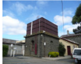
KYNETON RAILWAY STATION COMPLEX SOHE 2008
