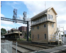
KYNETON RAILWAY STATION COMPLEX SOHE 2008
