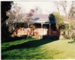
Wingrove Cottage Pines 672 674 Main Rd Colour 3 - Shire of Eltham Heritage Study 1992
