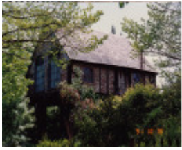
Jarrold Cottage Shop Studio 701 Main Rd Colour 2 - Shire of Eltham Heritage Study 1992
