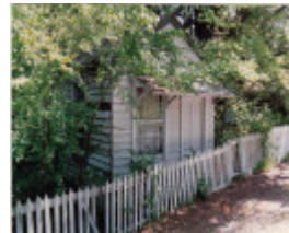
Jarrold Cottage Shop Studio 701 Main Rd Colour 1 - Shire of Eltham Heritage Study 1992
