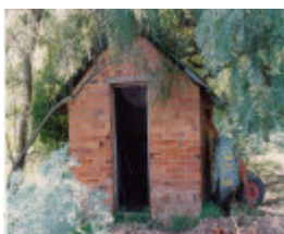
Living Learning Centre 739 Main Rd Eltham Colour 3 - Shire of Eltham Heritage Study 1992
