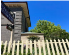
2023. 1905 'lean to' addition occupies the footprint of original conservatory.
