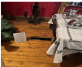
2023. Subfloor bank vault locking mechanism in dining room of the first floor, connects to the bank vault below.
