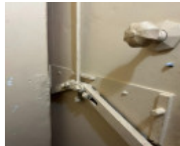
2023. Bank vault locking mechanism to ground floor.
