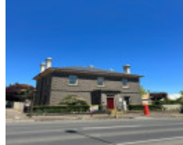
2023. Primary facade of Bank of NSW to Piper Street.
