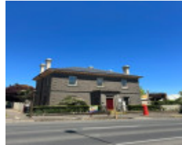
2023. Primary facade of Bank of NSW to Piper Street.
