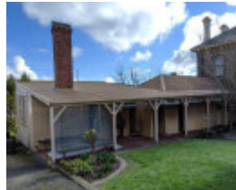
2023. Washhouse, kitchen and southern elevation of bank building.
