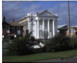
1 former baptist church ballarat front view
