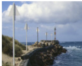
new works lakes entrance view of barrier
