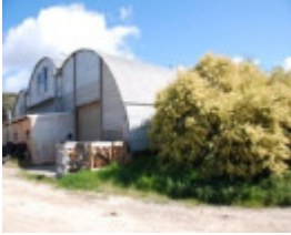
B5438 Former Quonset Hut
