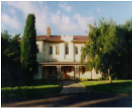
B6939 Farm Workers Block
