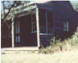
New Works cottage
