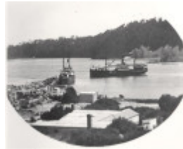
New Works, Lakes Entrance
