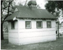
B3712 Former Cab-Man's Shelter
