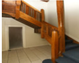
B4908 Canterbury Mansions Entrance Stairway
