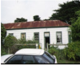
1 former wattle hill hotel lavers hill front view april 1994
