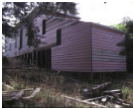
former wattle hill hotel lavers hill rear view april 1987
