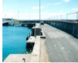
B6494 Fisherman's Breakwater North View
