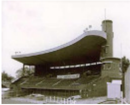
B6353 Glenferrie Sports Ground Grandstand
