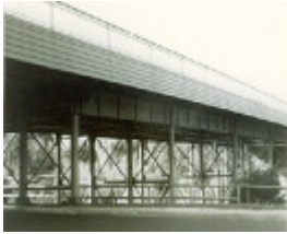
B1600 Metal Truss Bridge
