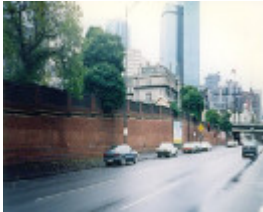
B6442 Retaining Wall
