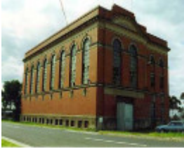
B3682 Albion Sub-Station
