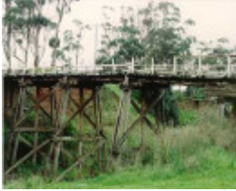
B3737 Trestle Bridge Keilor
