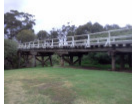
B3737 Trestle Bridge Keilor 2012
