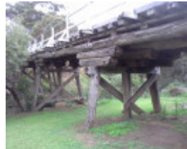
B3737 Trestle Bridge Keilor
