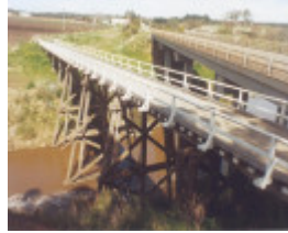
B3737 Trestle Bridge Keilor
