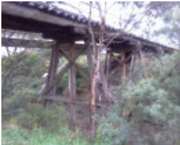
B3737 Trestle Bridge Keilor
