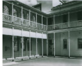
B2536 Former Mount Royal Geriatric Hospital, 36 - 56 Poplar Rd, Parkville
