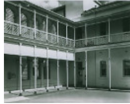
B2536 Former Mount Royal Geriatric Hospital, 36 - 56 Poplar Rd, Parkville
