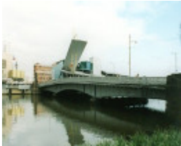
B6799 Spencer Street Bridge
