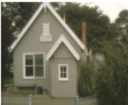
little hampton primary school no 1700 side view
