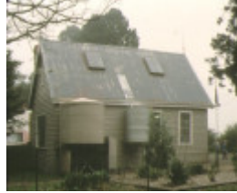
little hampton primary school no 1700 rear view
