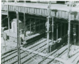
B3120 Swanston St Bridge Over Rail Lines
