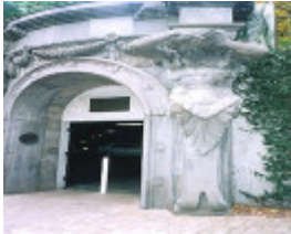
B6479 Underground Carpark
