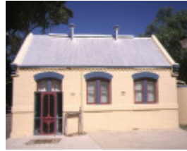
1 primary school no 744 lockwood front view dec1997
