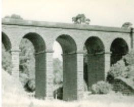
B1787 Railway Viaduct, Sunbury
