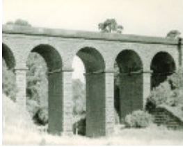
B1787 Railway Viaduct, Sunbury
