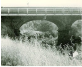
B3039 Bluestone Road Bridge
