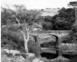
B0910 Bluestone Bridge
