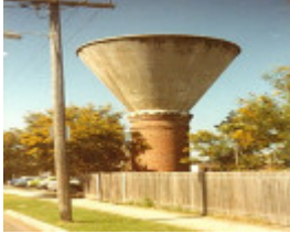
B5123 Water Tower
