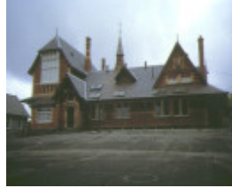
former primary school number 2120 long gully rear view
