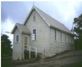
former primary school number 2120 long gully timber classroom
