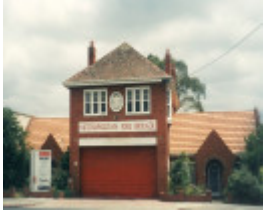
B6894 Fire Station
