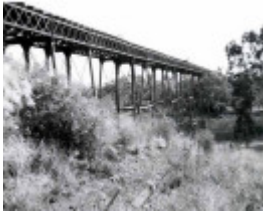
B3741 Railway Viaduct Melton
