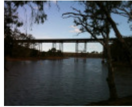
B3741 Melton Viaduct Railway Bridge
