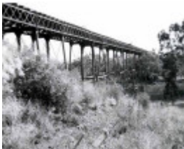
B3741 Railway Viaduct Melton
