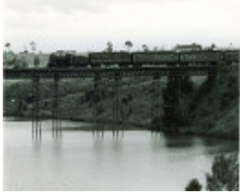
B3741 Viaduct Railway Bridge
