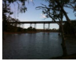
B3741 Melton Viaduct Railway Bridge
