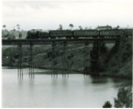
B3741 Viaduct Railway Bridge
