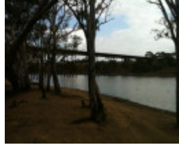
B3741 Melton Viaduct Railway Bridge
