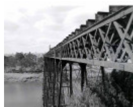
B3741 Railway Viaduct Melton
