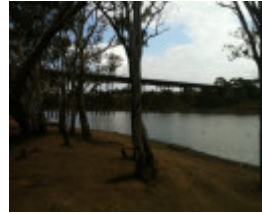
B3741 Melton Viaduct Railway Bridge
