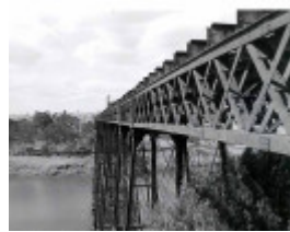
B3741 Railway Viaduct Melton
