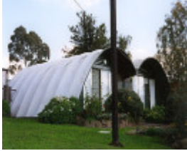
B4835 Former Supermarket
