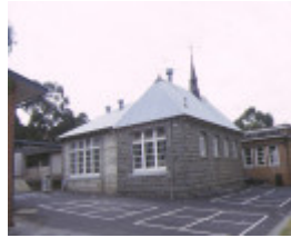
1 primary school no 2162 grove road lorne yard view mar1998
