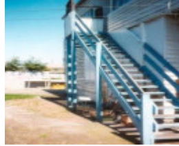
B7110 Outside Stairs
