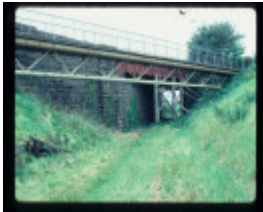
RAILWAY BRIDGE AND CUTTING
