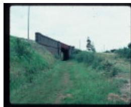
RAILWAY BRIDGE AND CUTTING
