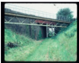
RAILWAY BRIDGE AND CUTTING
