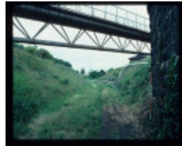
RAILWAY BRIDGE AND CUTTING
