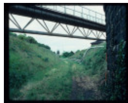
RAILWAY BRIDGE AND CUTTING
