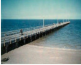
B3436 Kerferd Rd Pier Albert Park
