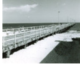
B3436 Kerferd Rd Pier
