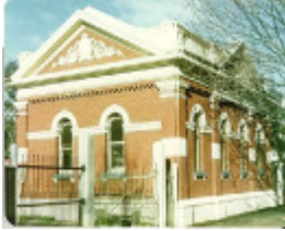
B4602 Gas Valve House
