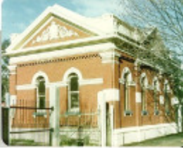
B4602 Gas Valve House
