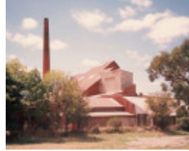
B5992 Box Hill Brickworks
