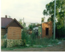
B5992 Box Hill Brickworks
