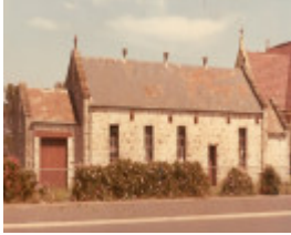
B4315 Former St Andrew's Catholic Church
